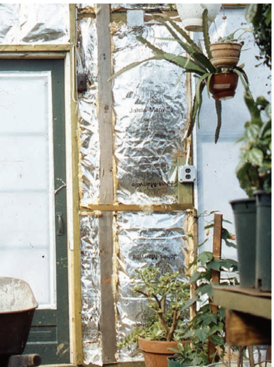
Top: Insulation board or aluminum foil can reduce the wall temperature behind sidewall heat pipes by as much as 40° F. Bottom: Insulating the north wall of the greenhouse, although it saves energy, reduces the reflected light from clouds and snow.
